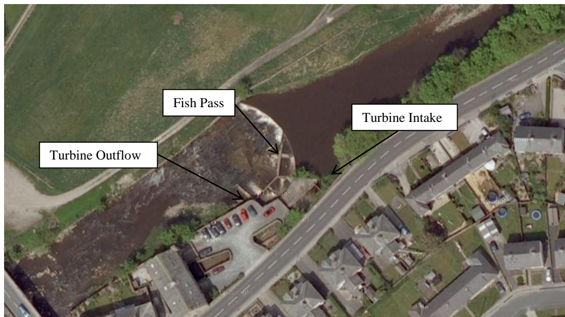
Figure 2.1. Settle Hydro Site with the location of the turbine intake and outflow and fish pass detailed. © The GeoInformation Group. Accessed Google.co.uk, 14/12/12.
